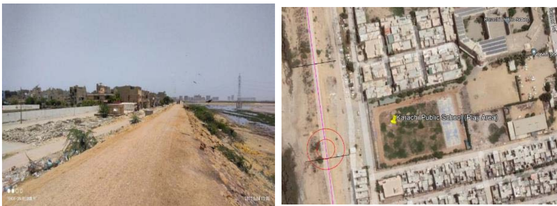
Interceptor Alignment on the Right beyond the retaining wall and Karachi Public School (Play Area) Boundary Wall on the Left
