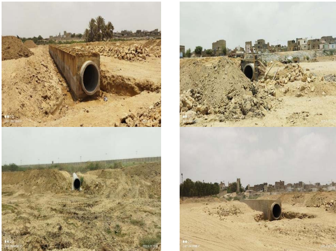
Figure 3-21: Sewer Culverts in Malir Expressway Alignment
