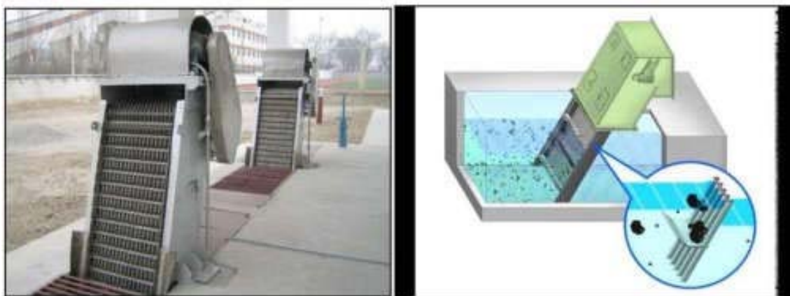
Figure 3-10: Typical View of Coarse Screens
