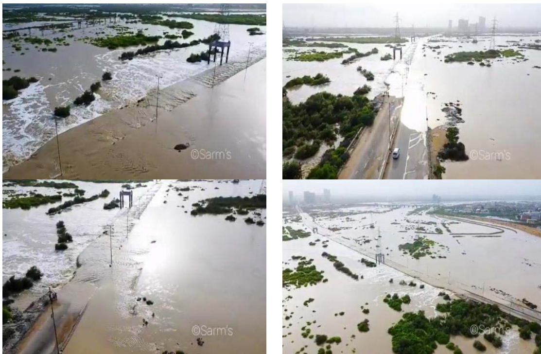
Figure 4-6: Flood Situation at Korangi Crossing Road (27 July 2022)
