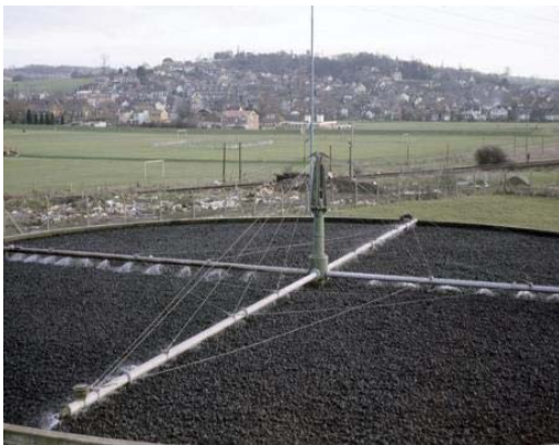
Figure 3-14: Typical View of Trickling Filter Unit
