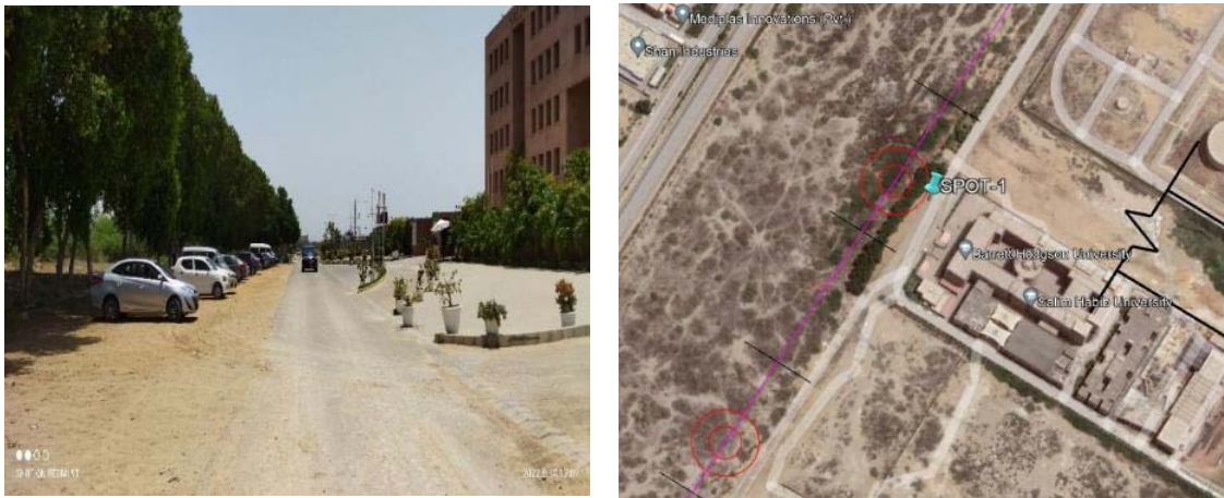
Interceptor Alignment on the Left beyond the Tree Line and Salim Habib University on the Right
