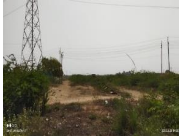
One of the Dhabeji Rising Main Lines near N5 National Highway
