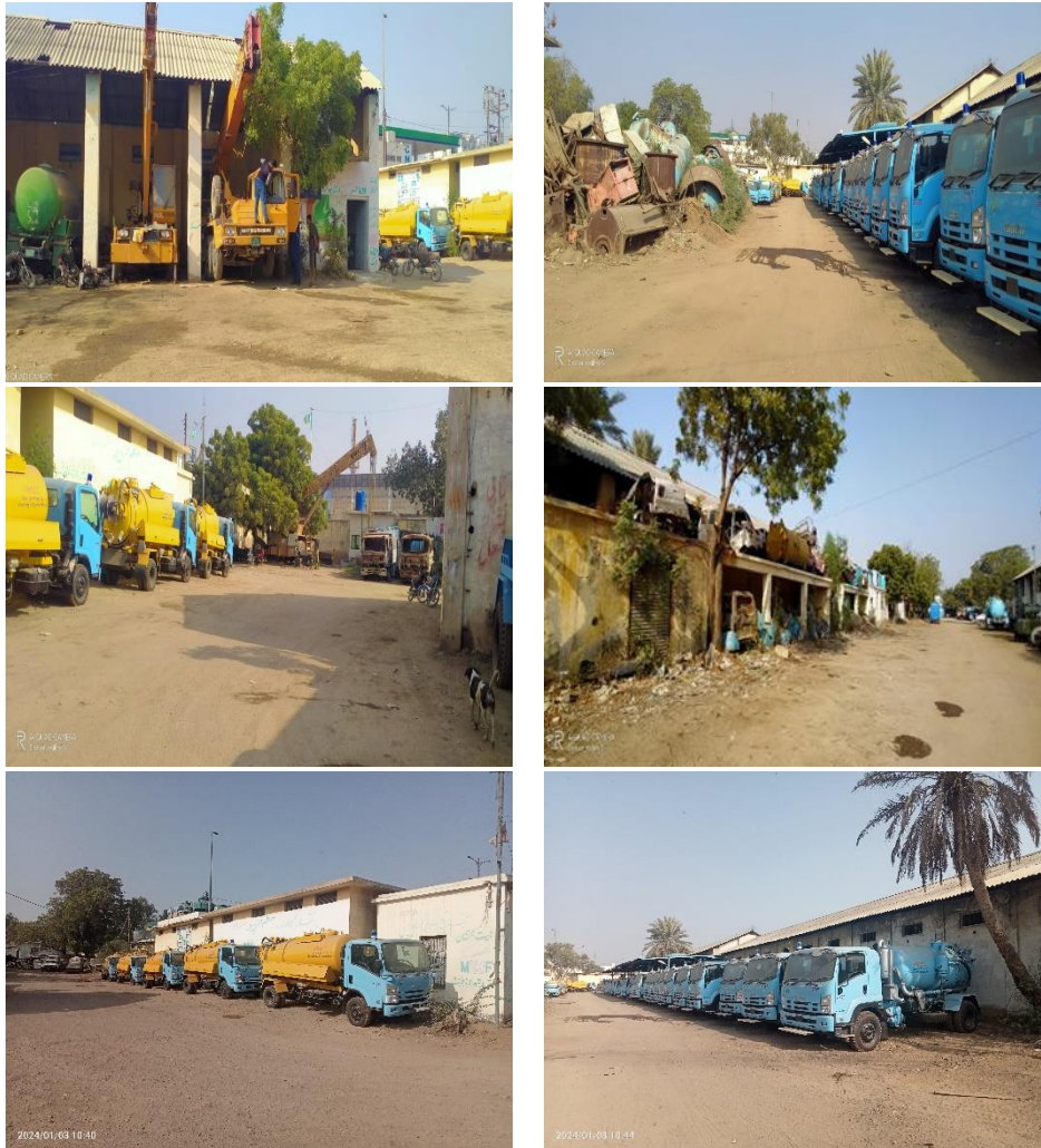
Plate 2.1: Existing Site Conditions SCE&S Division at KW&SC Central Workshop at 9th Mile
