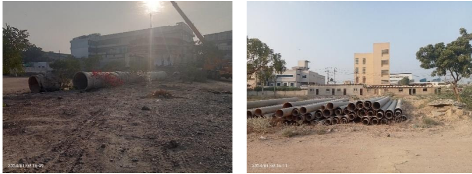
Plate 2.2: Existing Site Conditions PS-II Site at Korangi
