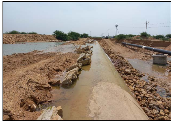
Exposed portion of G.K Conduit along Creek-1 – From Right Bank
