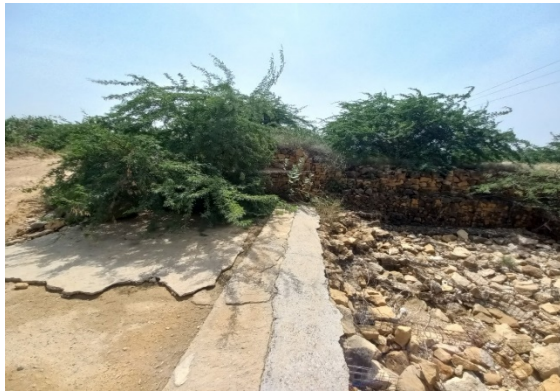
Existing Condition of Stone Protection in Creek-2
