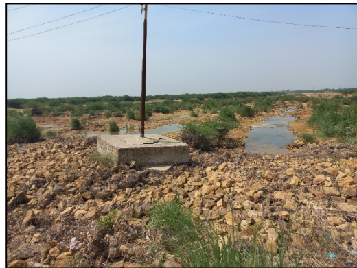
Exiting Stone Protection at Downstream of Pipeline Corridor
