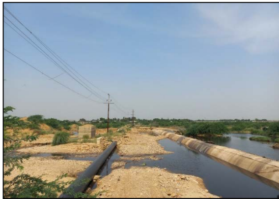
Exposed portion of G.K Conduit along Creek-1 – From Left Bank
